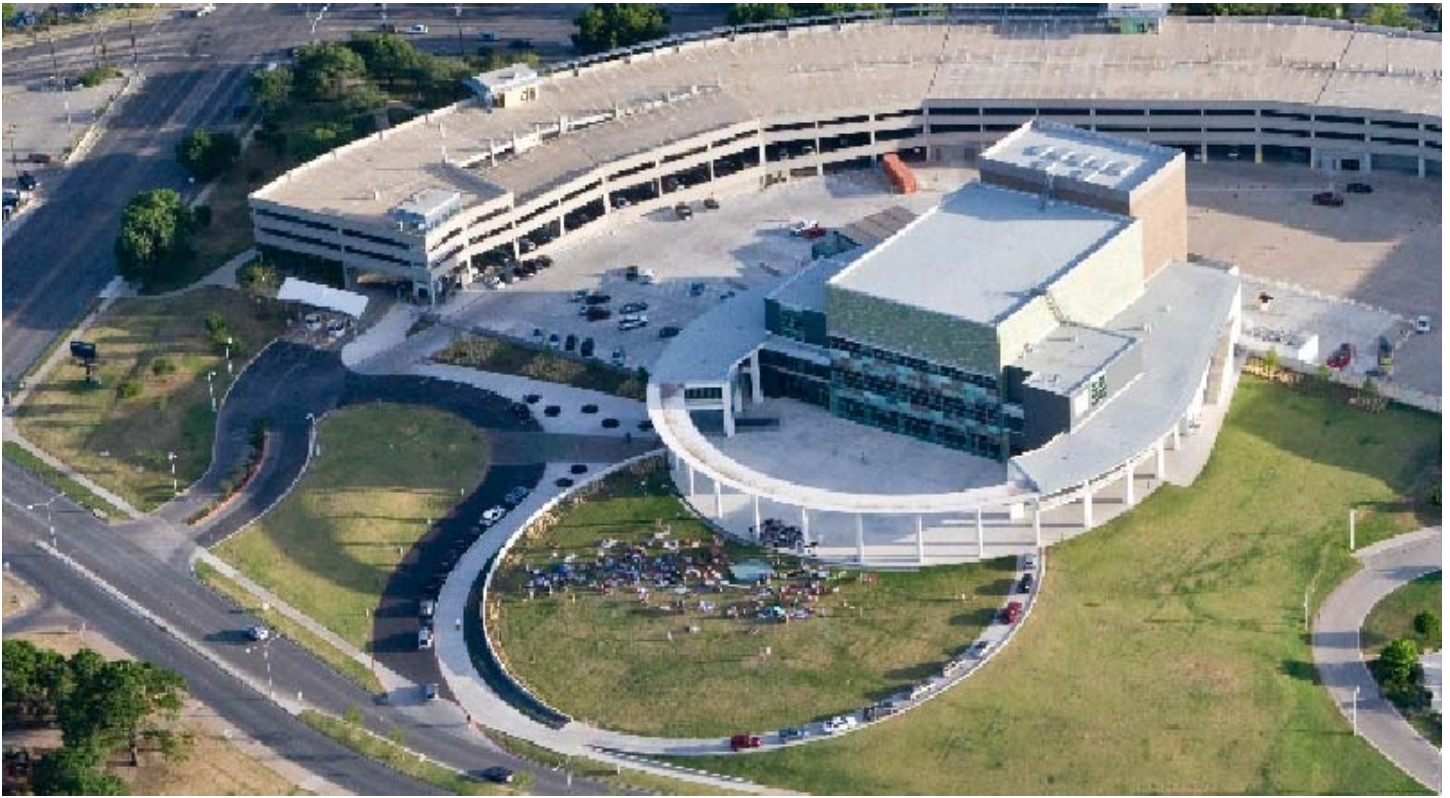
Aerial photo of The Long Center & Palmer Events Center Parking Garage
